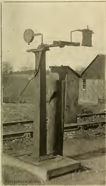
STATION PILLAR SET READY FOR EXCHANGE.
